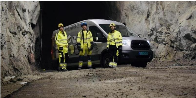
Manon (left) and her colleagues in a mine in Odda (Norway) performing well logging to define the hydraulic conductivity of the formation to define the potential of waste storage in the mine.
